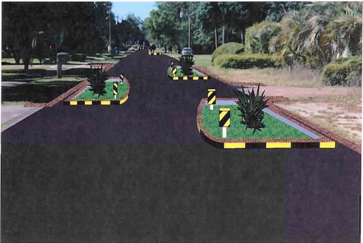
Figure 8. Chicane Installation on Country Club Avenue
