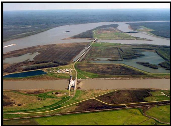
Figure 5. Corps of Engineers Old River Control Structure north of Baton Rouge, LA. Mississippi River leftside and Atchafalaya River on the rightside.
